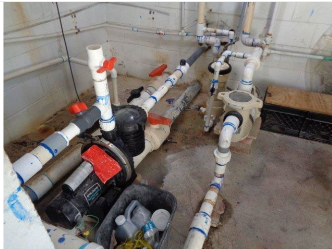
138. Inground pool pumps and filter.
