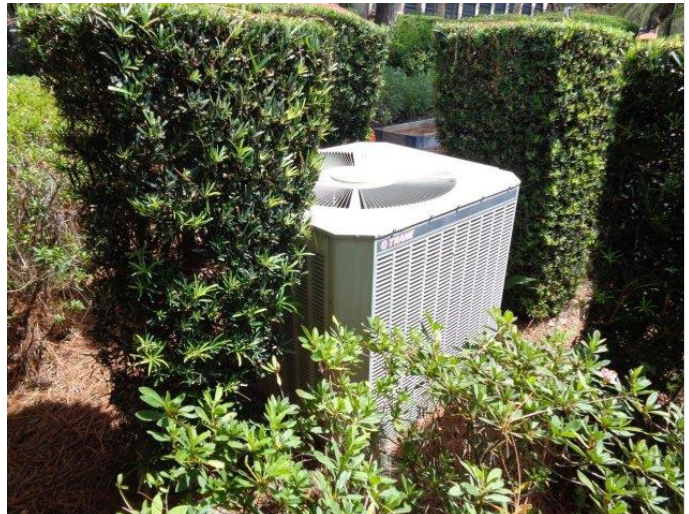
111. Typical split system a/c condenser at grade.
