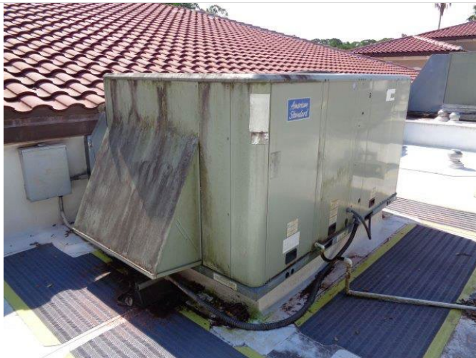
114. Typical packaged RTU.
