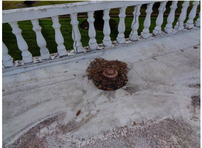
98. Typical interior roof drain. Note the debris partially blocking the drain strainer.
