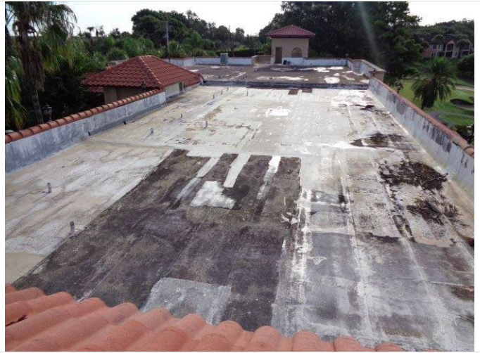
86. Partial view of the roof atop the San Diego building, looking east. Note the BUR membrane.
