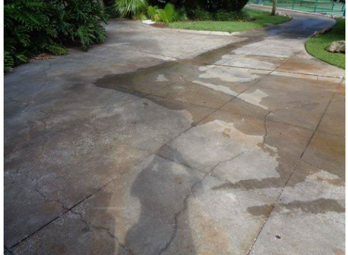
26. Patio area between the San Miguel and San Diego buildings. Note the cracks in the concrete sidewalk.
