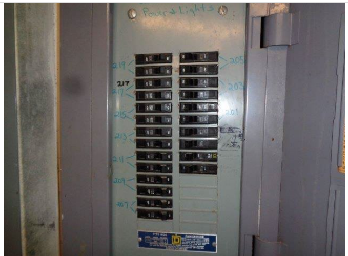
125. Typical distribution panel for the individual guestrooms.
