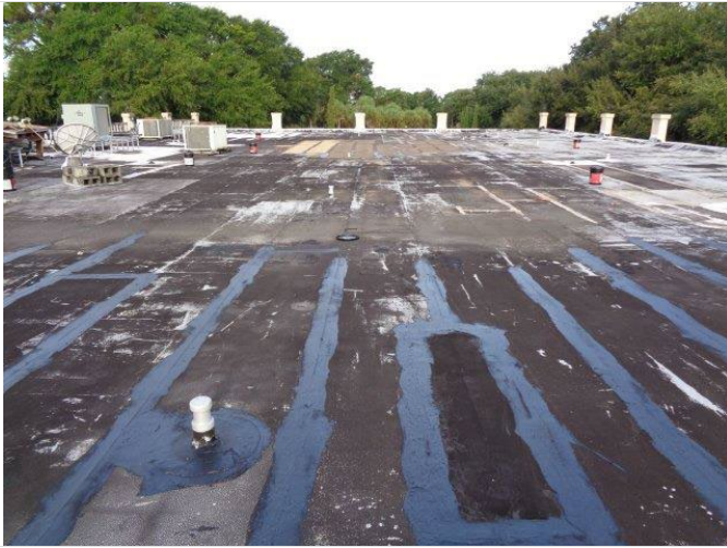
91. Partial view of the roof atop the Conference Center building, looking west. Note the BUR membrane.
