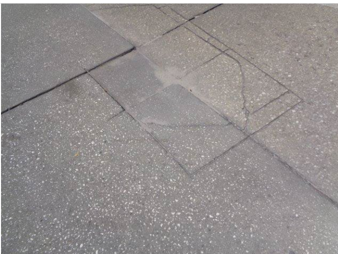
29. Flatwork at the south end of the Golf Club. Note the tripping hazard.
