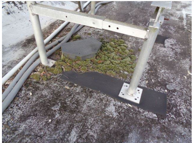
104. Moss was observed below one of the RTU's atop the Convention Center roof.
