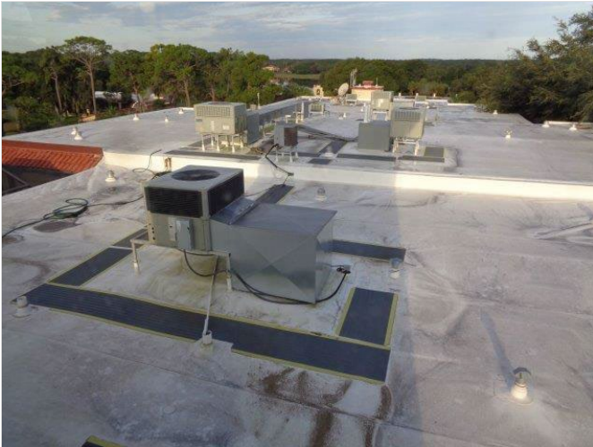
108. Typical packaged RTU's and a/c condensers atop the roof.
