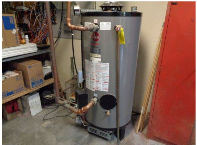
135. Typical individual domestic hot water heater.
