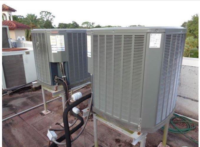
109. Typical split system a/c condensers atop the roof.
