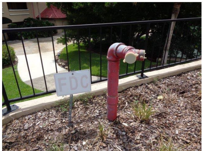
197. Typical fire department connection.
