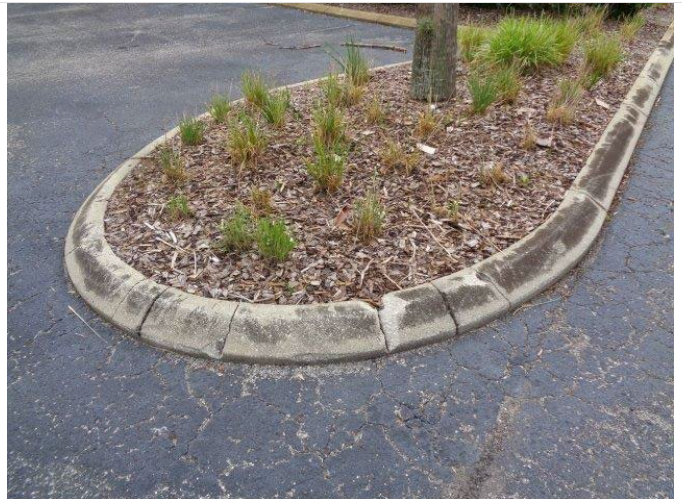
22. Typical cast-in-place concrete curb damage.
