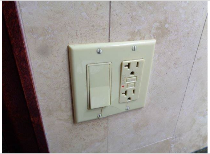
127. Typical GFCI outlet.
