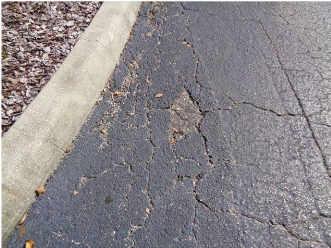
21. Typical asphalt pavement damage.
