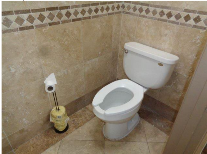
200. ADA designated stall does not meet maneuverability requirements of 60" diameter radius.
