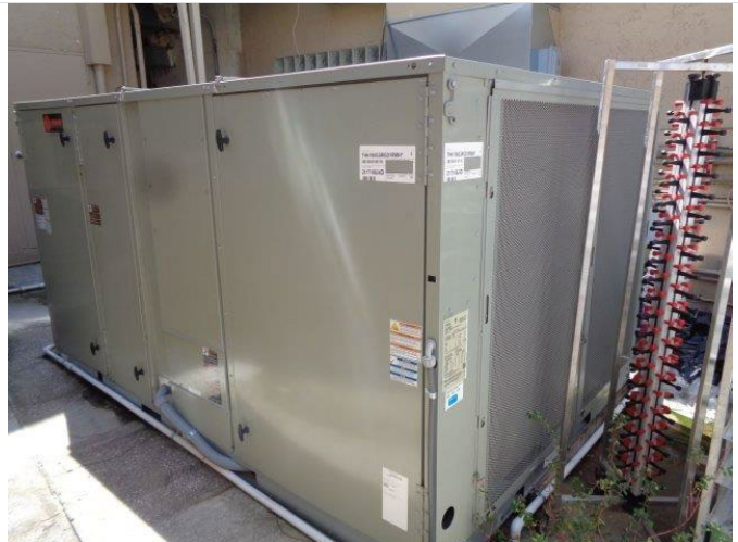
117. New packaged 10-20 ton unit behind the Restaurant Complex.
