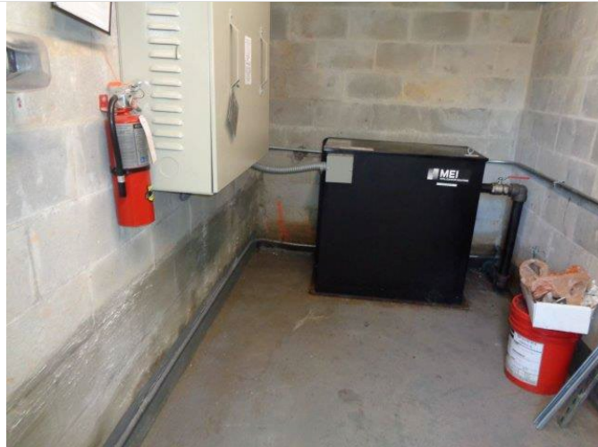
144. Typical hydraulic elevator equipment.
