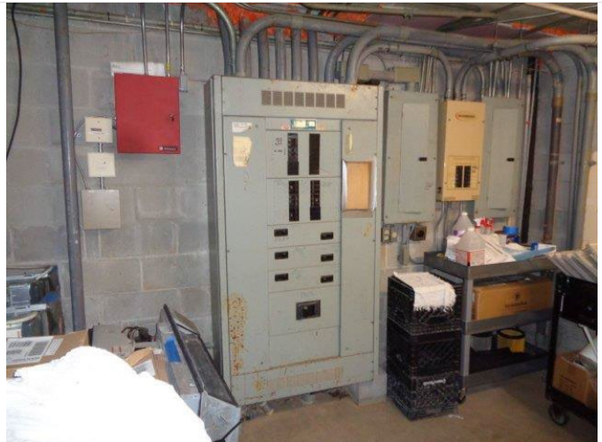
123. Typical main electric panel and distribution panels.
