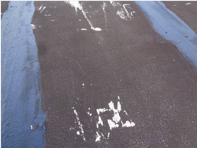
99. Typical BUR membrane damage.
