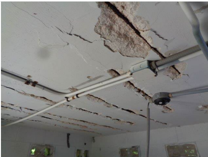
59. Spalled concrete and corroded rebar in the concrete shed referenced in Photo 58.
