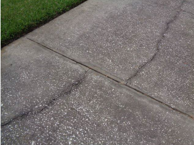
25. Typical cracks in the concrete sidewalk.
