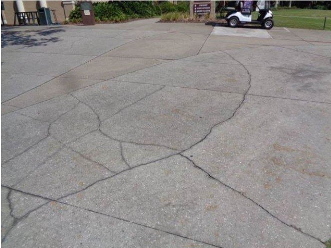
27. Patio area at the south end of the Golf Club. Note the cracks in the concrete sidewalk.
