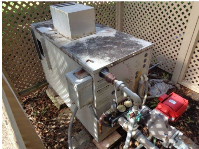
131. Typical gas-fired hot water boiler for the Resort Hotel.
