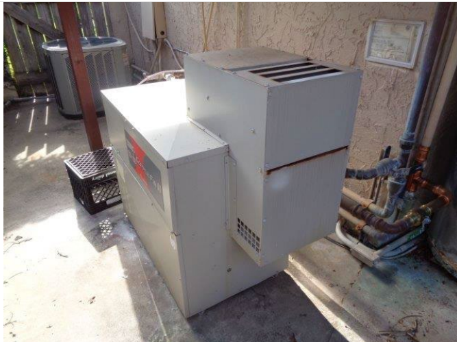
132. Typical gas-fired hot water boiler for the Resort Hotel.
