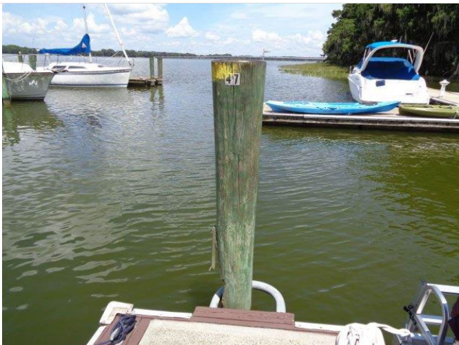
65. Typical wood pier foundation for the concrete slips.
