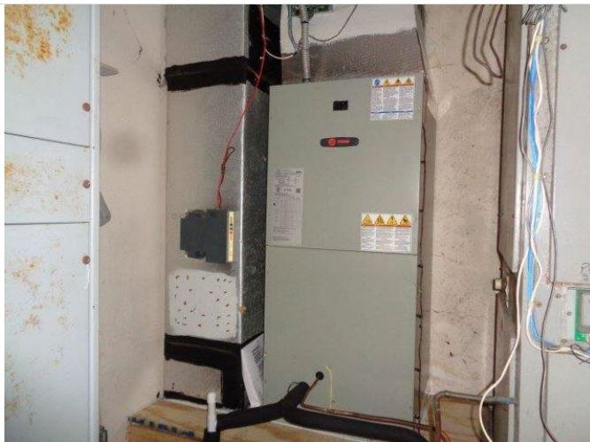
118. Typical split system furnace.
