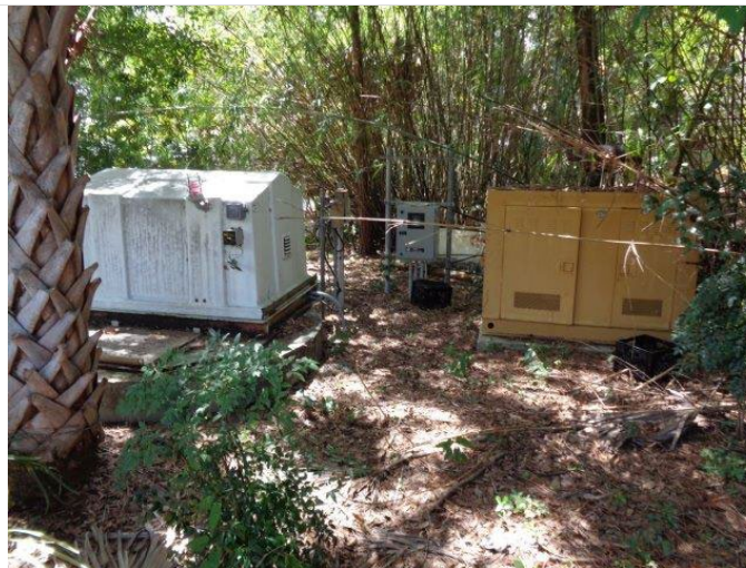
130. Diesel emergency electrical back-up generator for the lift station at the Resort Hotel.
