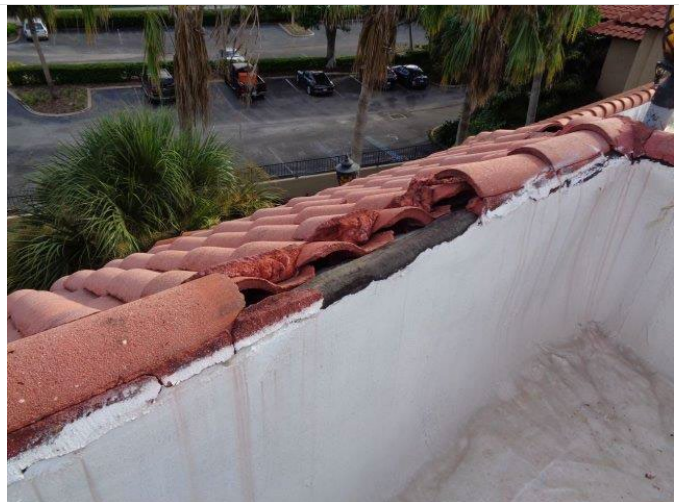
102. Damaged clay terracotta coping.
