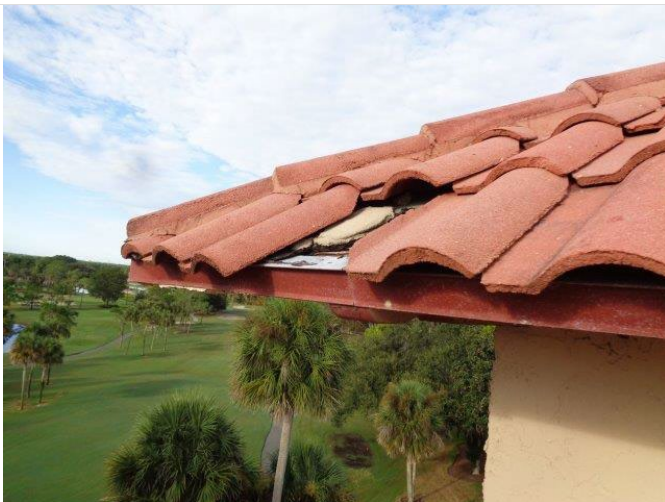
101. Damaged clay terracotta tile.
