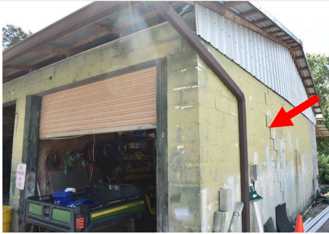
198. South side of one of the landscaping buildings. Note the step crack in the CMU wall.
