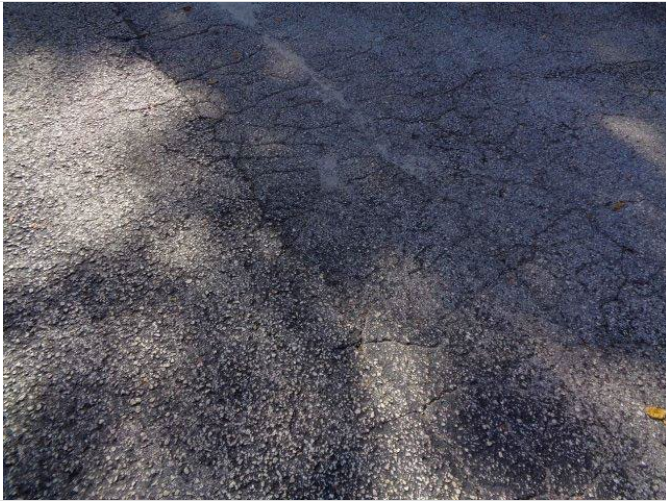
19. Typical asphalt pavement damage.
