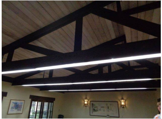
56. Typical wood truss roof framing.
