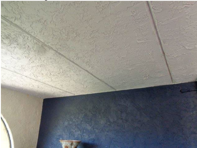
51. Typical precast concrete plank floor framing in the Resort Hotel buildings.
