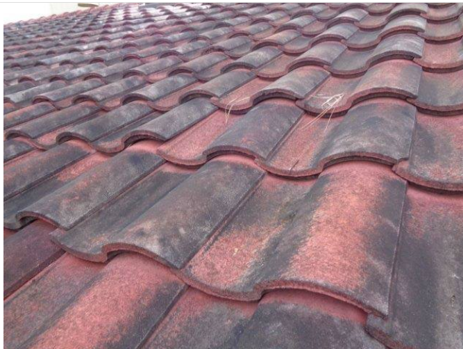
103. Stain terracotta tiles. Note that this does not effect the water shedding capability of the tile.
