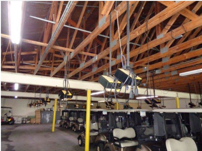
57. Typical wood truss roof framing in the Golf Club parking garage.
