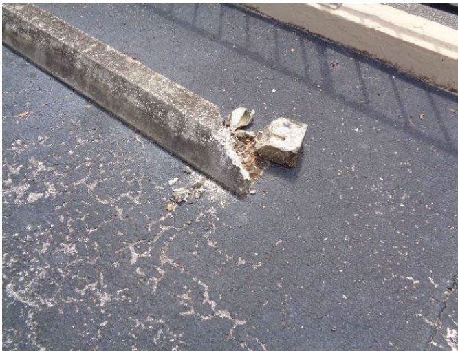
23. Typical damage to a precast concrete wheelstop.
