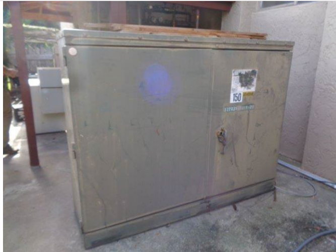
120. Pad mounted electrical transformer at the Resort Hotel.
