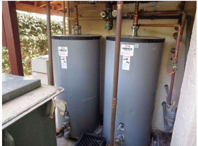
133. Typical hot water storage tanks for the Resort Hotel.
