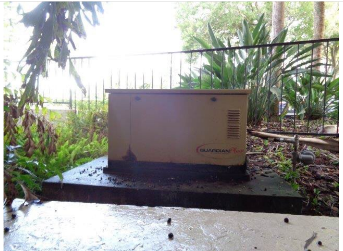
129. One of two natural gas emergency electrical back-up generators at the Resort Hotel.
