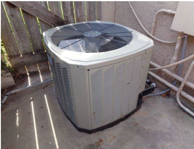
110. Typical split system a/c condenser at grade.
