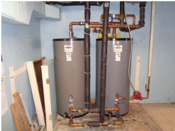
134. Typical hot water storage tanks for the Resort Hotel.
