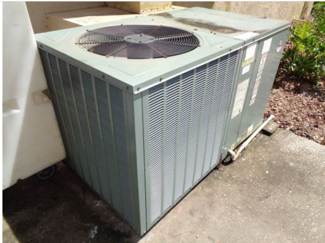
116. Typical packaged unit at grade.
