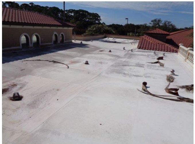
96. Partial view of the roof atop the Golf Club, looking south. Note the TPO membrane.
