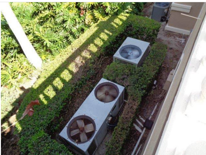
112. Typical packaged unit at grade.
