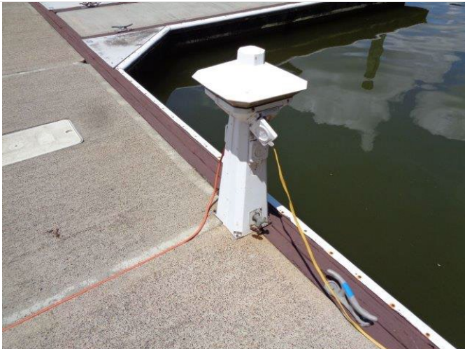
188. Typical shore power station for the Marina slips.
