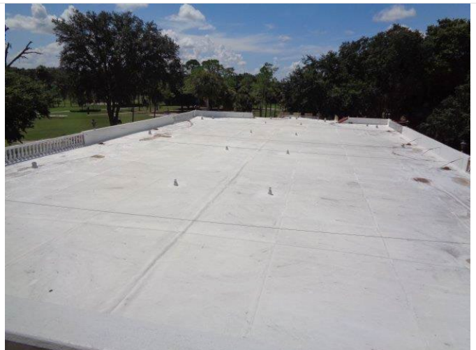
90. Partial view of the roof atop the San Angel building, looking south. Note the TPO membrane.
