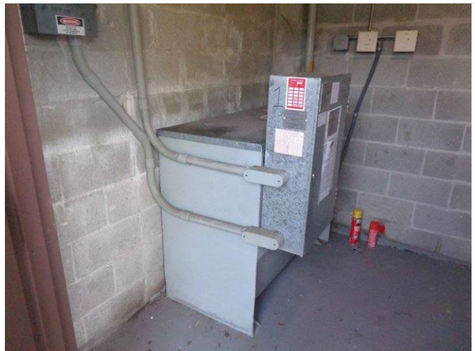
143. Typical hydraulic elevator equipment.
