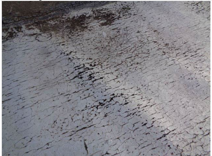
100. Typical BUR membrane damage.
