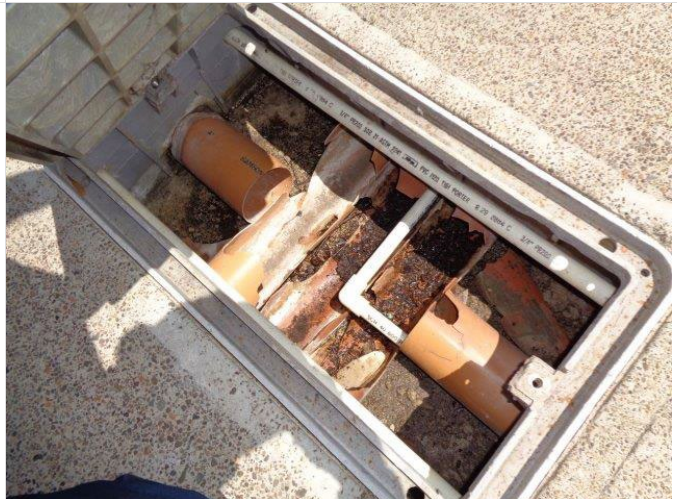
189. Typical access panel for the boat slips. Note the damaged/deteriorated electrical passthrough tubes.
