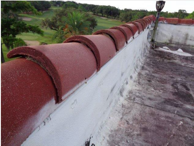
97. Typical parapet wall atop the roof.
