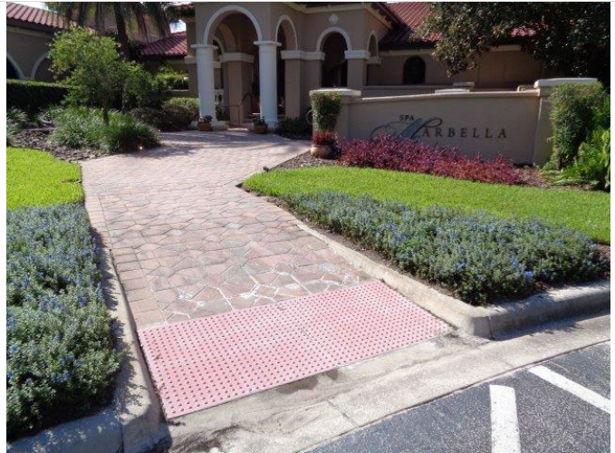
38. ADA traction pad at the curb cut to the main entrance of Spa Marbella.
