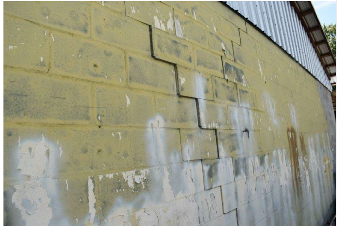
199. Close up view of the step crack referenced in Photo 198.
