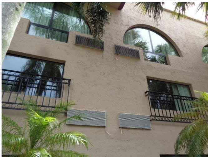
107. Through wall louvers for the typical PTAC unit of the guestrooms.
