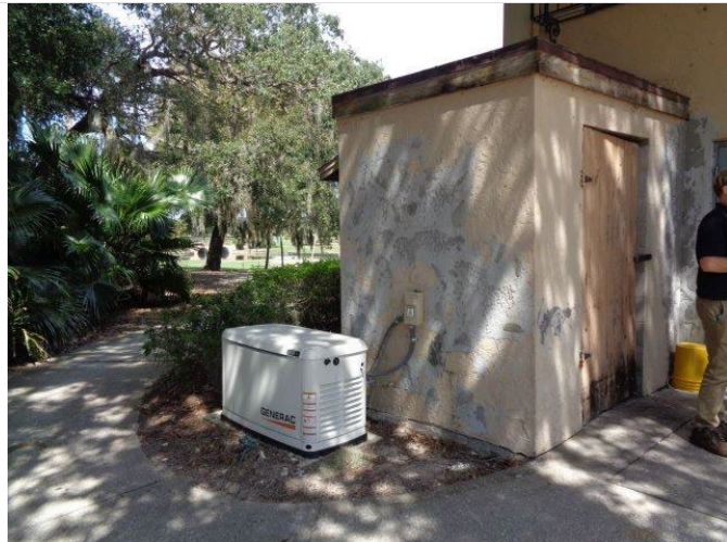
128. One of two natural gas emergency electrical back-up generators at the Resort Hotel.
