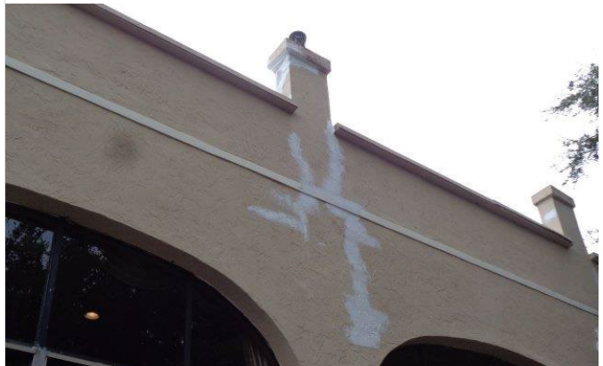
76. Closer up of the north façade referenced in Photo 75. Note the stucco repairs.
