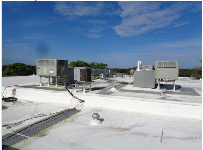
88. Partial view of the roof of the San Miguel building. Note the TPO membrane and various RTU's and a/c condensers.
