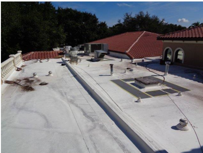
95. Partial view of the roof atop the Golf Club, looking north. Note the TPO membrane.
