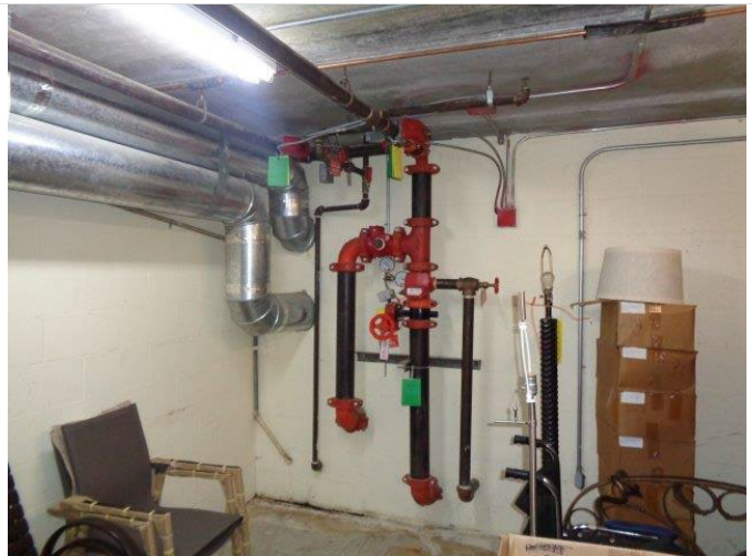
193. Typical fire sprinkler riser in the Resort Hotel.
