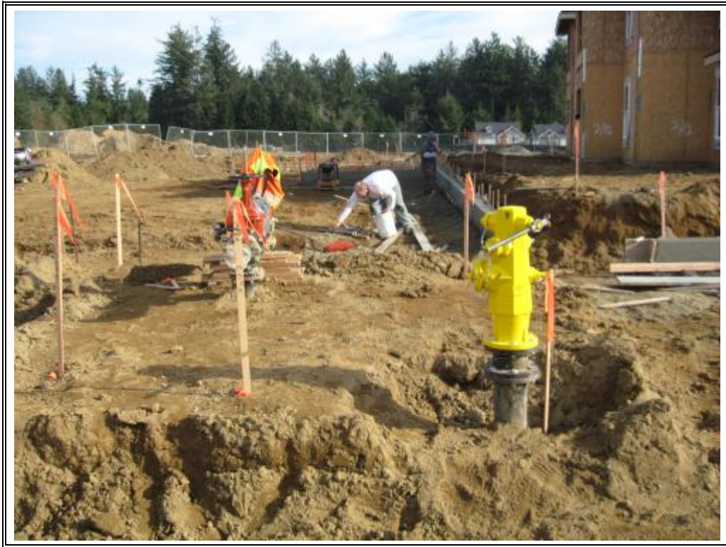
11. Fire hydrant and curb/gutter forms at Building E.
