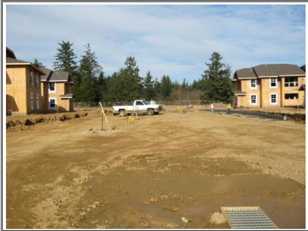
7. Access road and placing between buildings.
