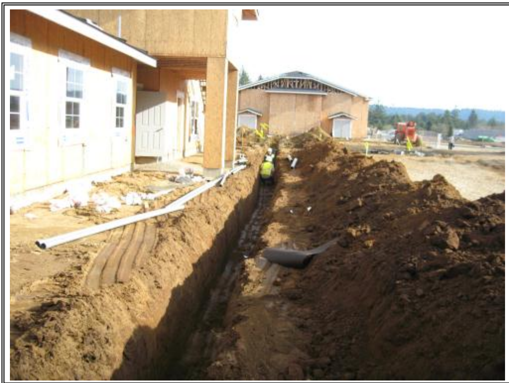
6. Underground electrical conduit installation.
