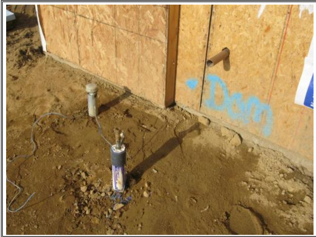
9. Water and gas stub to building.
