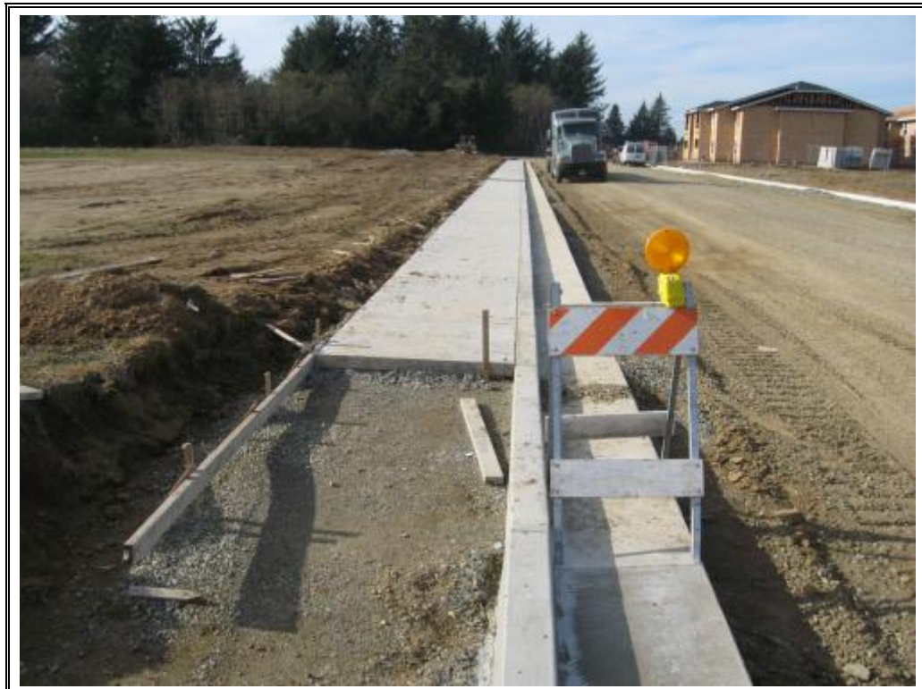
3. Curb, gutter and sidewalk at main entrance drive.
