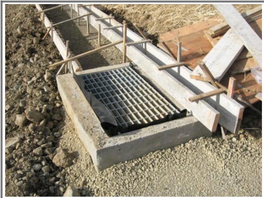
2. Storm drain inlet.
